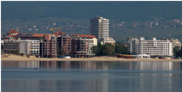
SUNNY BEACH: In April, on the eve of the summer tourist season, the resort was still dotted by construction sites, one of the main reasons for complaints by foreign tourists in recent years. Photo: Julia Lazarova
